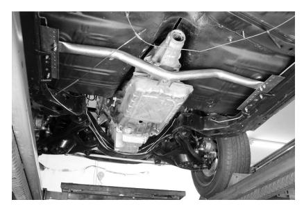
Install the crossmember frame brackets in the original factory bolt holes then mount the Crossmember. (64-67 convertible chassis shown here)
