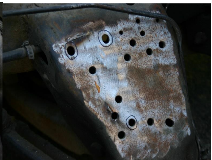
Passenger side holes
